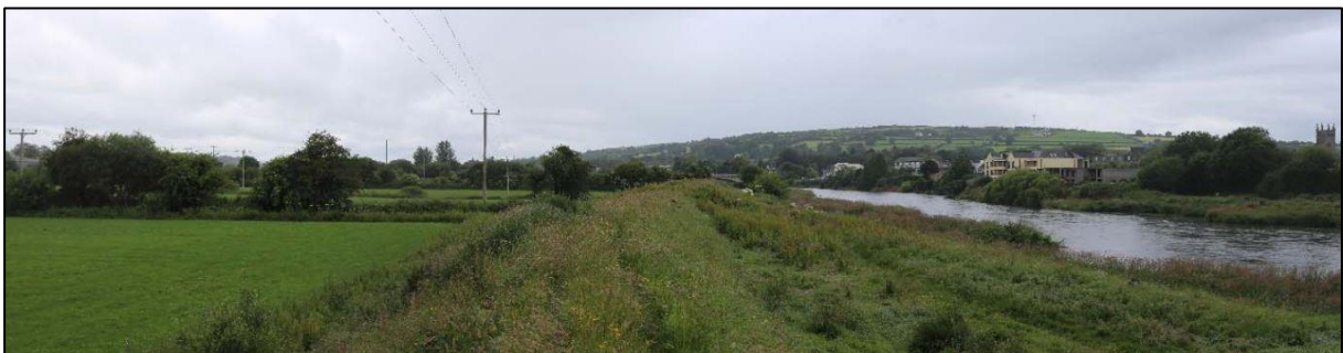
Figure 14-8: On bank of River Foyle, off site
